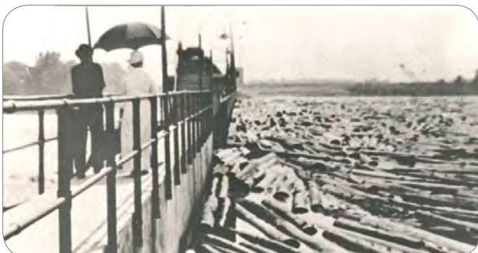
Coon Rapids Dam walkway open to pedestrians - note cut logs being transported. Source: Anoka County Historical Society
