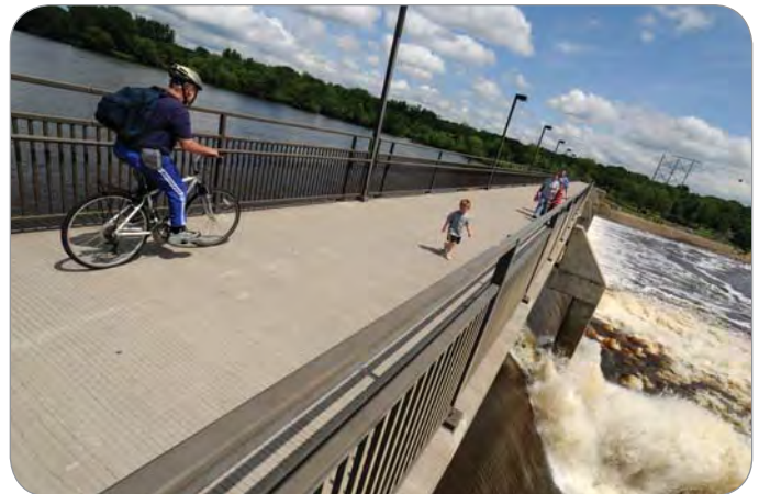
Coon Rapids Dam provides regional trail access across the Mississippi River.
