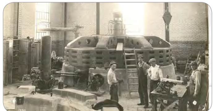
Coon Rapids Dam hydroelectric powerplant. Source: Anoka County Historical Society
