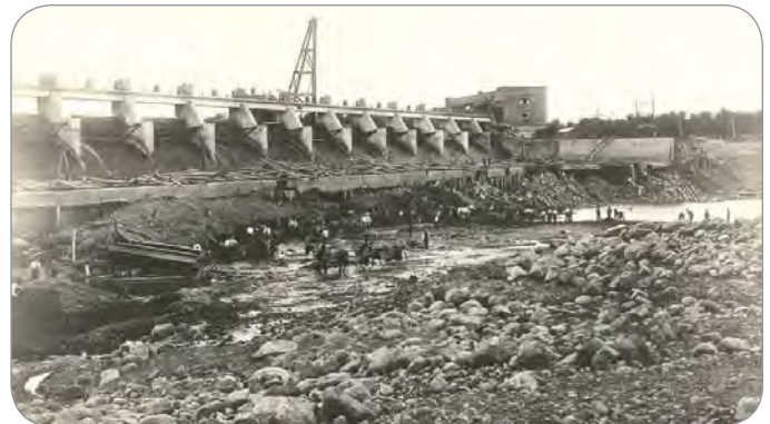
Coon Rapids Dam reconstruction nears completion. Source: Anoka County Historical Society
